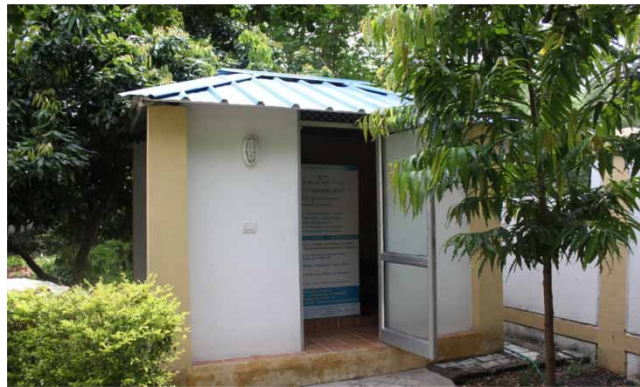
Figure 4 | ACFB System in XIDAS Priest Quarters.
